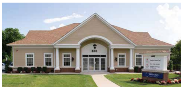
600 Montauk Highway, Suite C, Center Moriches
